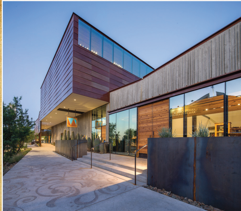
Western Spirit: Scottsdale's Museum of the West as seen from its northern perspective. Concrete walkways are imprinted with tooled leather designs inspired by Western saddles.
